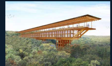
Iconic Zenbo Seinei building located in the forest
